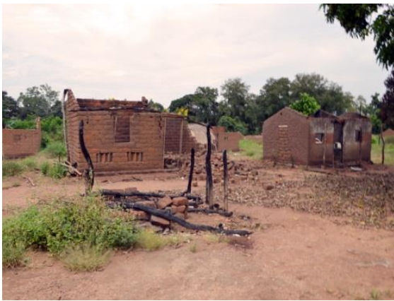
"Satisfactorily" rebuilt village clinic in BURP Project (Photo from Sara Imaji)
