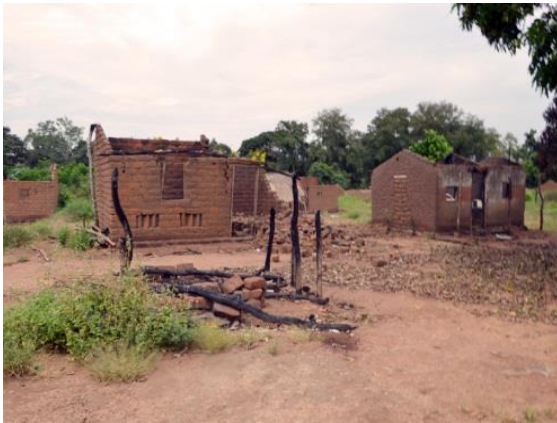
"Satisfactorily" rebuilt village clinic in BURP Project (Photo from Sara Emaji)
