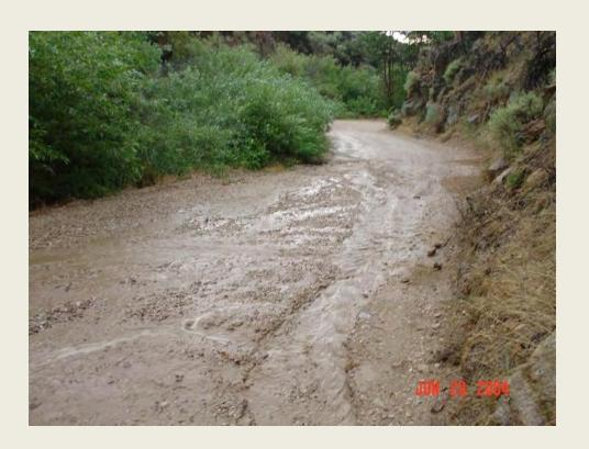
A stark illustration of the impact of inadequate drainage on a road surface...
